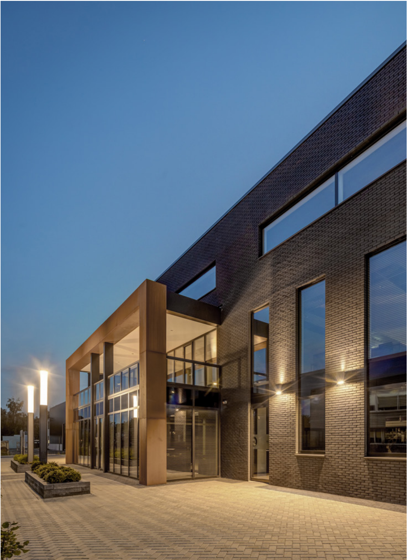
New building electrical wholesaler Robri | Wekerom | Netherlands
